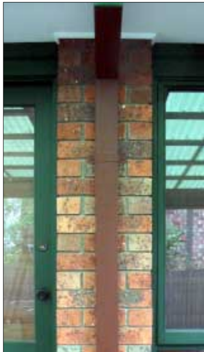
Before and after: the diverter simply fits into the downpipe.
