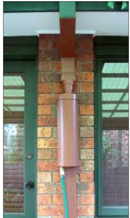
Before and after: the diverter simply fits into the downpipe.
